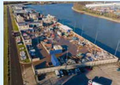
24 February Opening Dintelweg site
